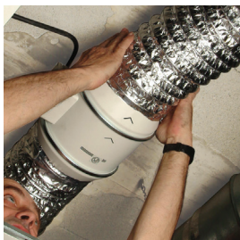
Connect the ducts.
