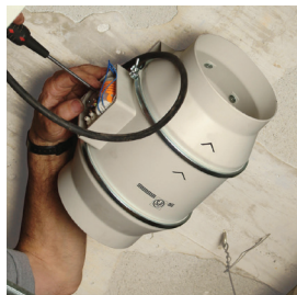
Carry out the wiring connections.
