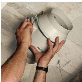
Place the impeller and motor.
