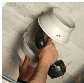
Fix the support bracket.
