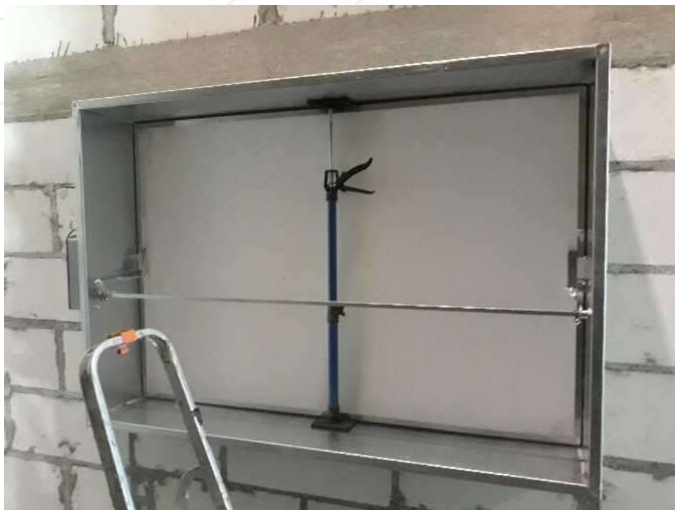
Figure 2. Correct preparation of the damper for installation (using spreader securing the housing)
