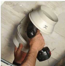
Fix the support bracket.
