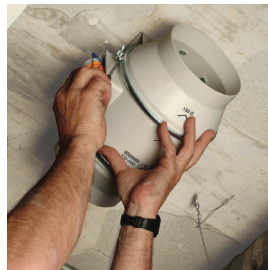
Place the impeller and motor assembly.
