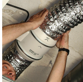
Connect the ducts.
